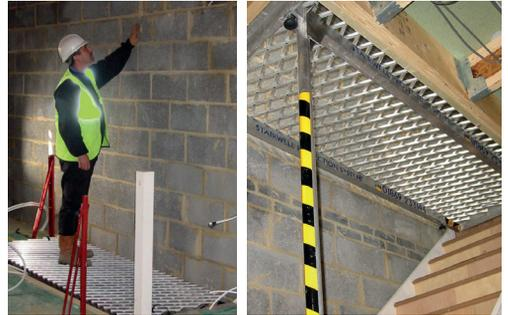
Safety Note: The mat is not suitable to be loaded out with materials. Maximum spread load is 225kg.
